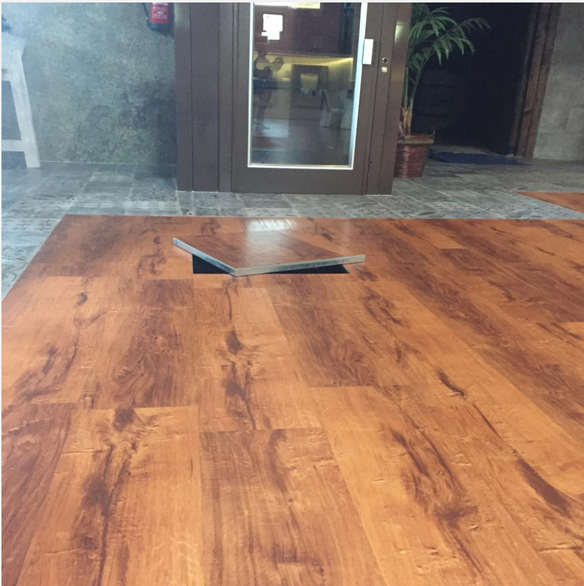
Laid on raised access floors.
